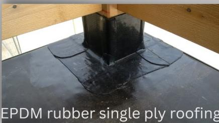
EPDM rubber single ply roofing
