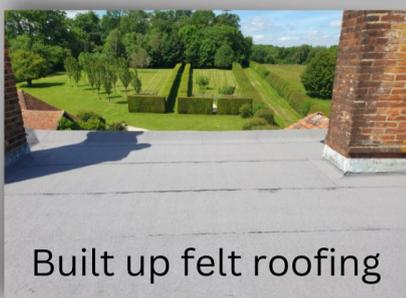
Built up felt roofing
